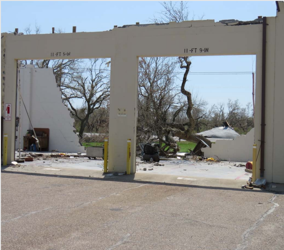
TxDOT's Rockport maintenance facilities
